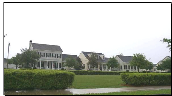
New Suburban Residential Development with Pedestrian Amenities
