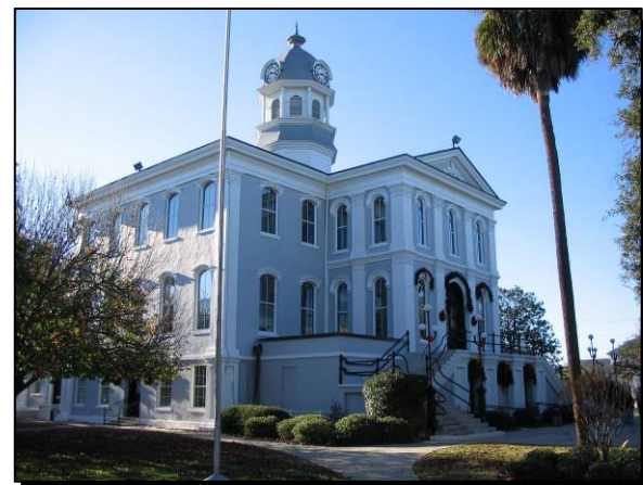
Representative Architecture for Institutional, County Courthouse
