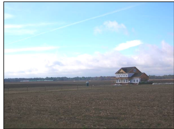
Rural Home in Thomas County
